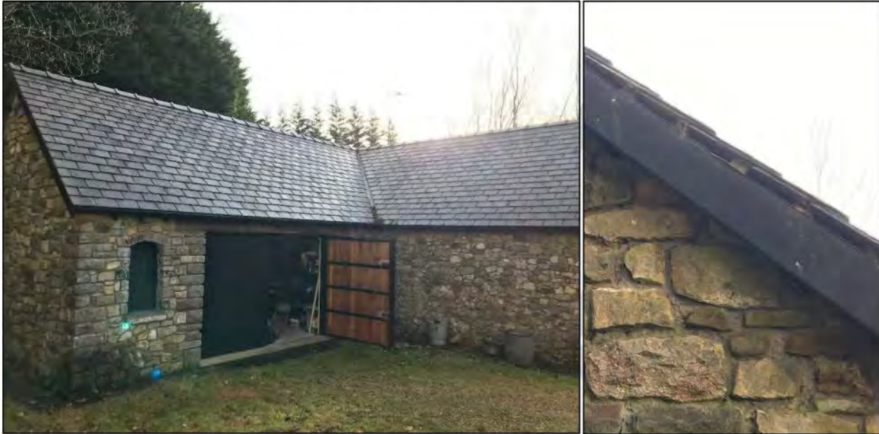
Plate 8 – Building 2: Converted Barn (left) with gaps under tiling (right)
